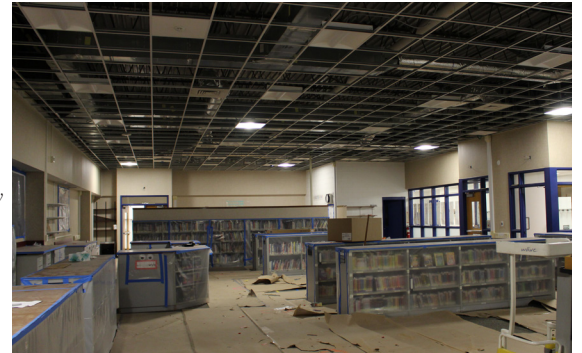
(right) Replacing ceiling and lighting at Park View library
