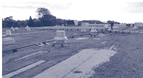
The roof at Glen Crest Middle School was installed in 1998. It needs frequent patches to keep water from leaking into the building. The coal tar/asphalt roof would be replaced by an energy-efficient rubber roof if the referendum is passed.
